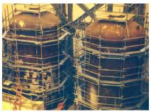
In order to remove the steam generators, pressurizer and reactor vessel, bio-shield walls had to be removed and an opening was required in the side of containment.
