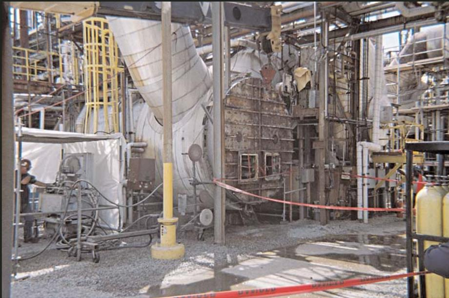
**Top:** Diamond wire sawing was used to cut the ends of a steel boiler at a chemical plant in Memphis, TN.
