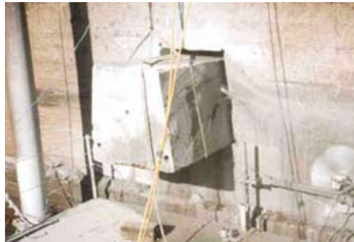
PLUG REMOVAL AT HYDROELECTRIC DAM
