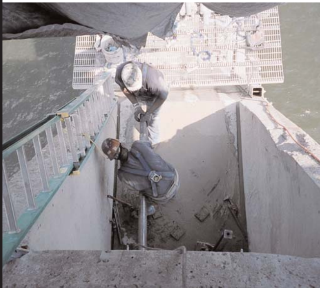
Left: Working inside the newly-created pocket, operators were tied off.
